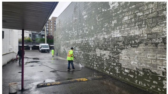
Surface prep on a commercial block wall before repainting.
