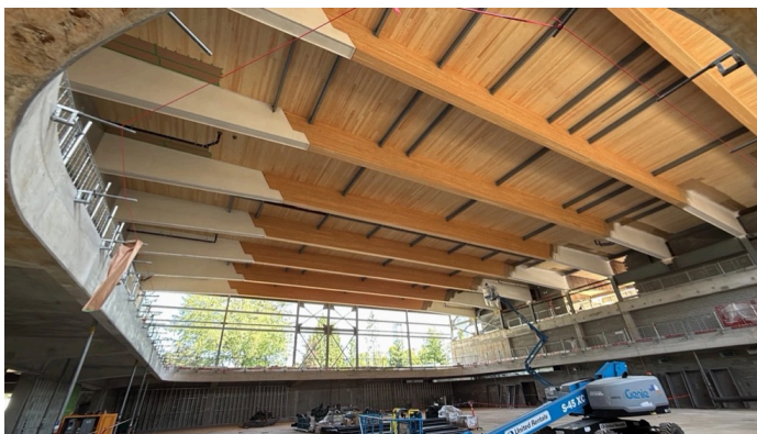
On site at a large commercial hall.
